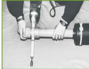
**10.** For warm up, the pipe and fitting are pushed onto the heating elements uninterrupted and without twisting. Push the pipe only up to the marked insertion depth and ensure that the marking remains visible during the warm-up time. The warm-up time starts after the welded parts have been pushed on completely.
