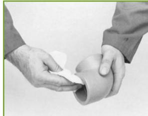
**06.** Clean the fitting by making circular movements over the entire internal welding surface of the fitting.
