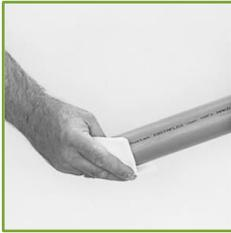
**04.** Clean the service pipes by using PB cleaner and tissues and make circular movements over the entire welding surface.
