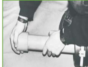
**11.** After the warm-up time has elapsed, the pipe and fitting must be pulled off the heating elements uninterrupted, without twisting and then inserted into each other until the weld bead on the pipe reaches the edge of the fitting. Minimal alignment of pipe and fitting is possible in the first 5 seconds. After that, steady the pipe and fitting for 1 minute (holding time). It is essential to observe the holding and cooling time.
