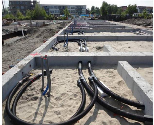
Figure 3: Alkmaar, NL: 6 houses connected to District Heating in 1,5 hrs
