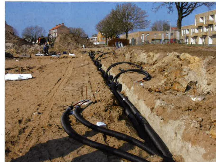
Figure 2. Installation of Flexalinks for new built houses
