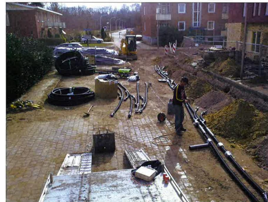
Figure 3. Laying of Flexalen with Flexalinks in the Klimopstraat
