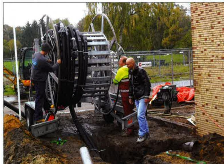
Figure 1. Uncoiling of 75 m Flexanet including ten house connections
