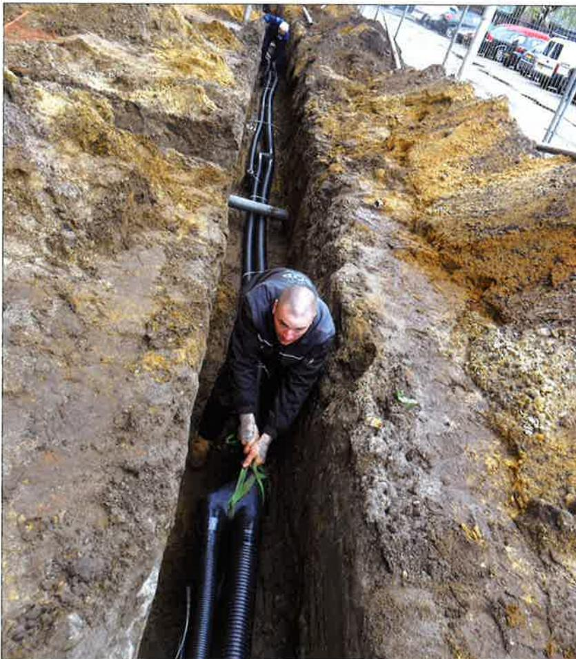
Figure 5. Pulling of the pre-fabricated network into the open trench – within 1,5 h the network was fully laid including all ten house connections
